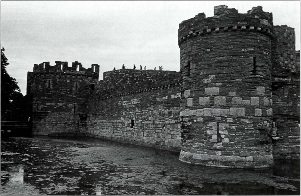
Tower 9, the adjacent curtain and the 'Gate next the Sea' beyond at Beaumaris. They all display light limestone on their lower courses but darker limestone above. (By kind permission of Anthony de Reuck)
