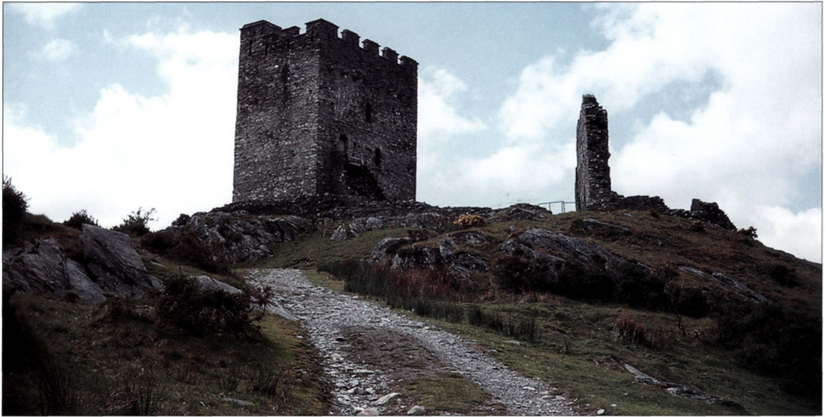
The square donjon of the Welsh castle of Dolwyddelan, built by Llywelyn the Great c.1221–40. After its capture, Edward I may well have added a storey to it but the battlements and line of mock drains are Victorian additions. The West Tower (to the right) may also be Edward's work.
