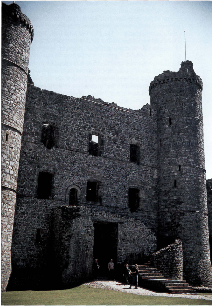
The great gatehouse at Harlech with its twin corner stair turrets, seen from the inner ward. The staircase wends its way up to the first floor hall door; the two halls (or chambers), each with a chamber on the left side, are marked by the large window openings.
