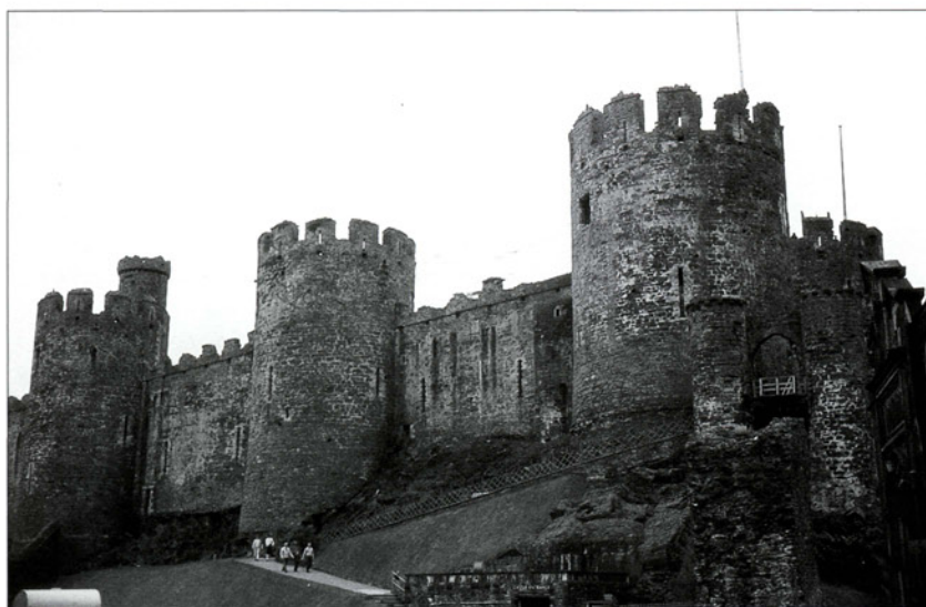
Conwy castle, begun in March 1283, from the north, showing the west barbican at the extreme left. The path is modern; originally entry was via a drawbridge spanning the pit in front of the small barbican bastions.
