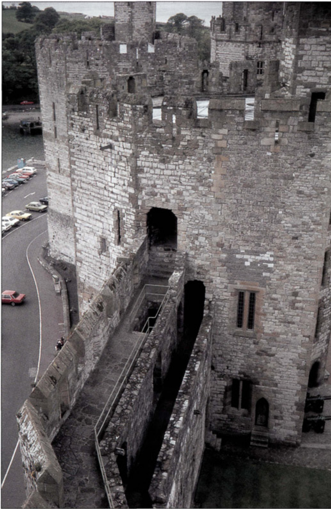
The Chamberlain Tower, with the Queen's Tower behind, seen from the Black Tower. The Chamberlain Tower on the south side once joined to the King's Gate on the north, thus demarking the Upper Ward from the Lower Ward beyond. The stair on the wall head leads down to the first-floor wall passage visible to its right; originally this would have been roofed over. Another passage runs below it at ground level. The kink in the walls marks where they cross the old Norman motte.
