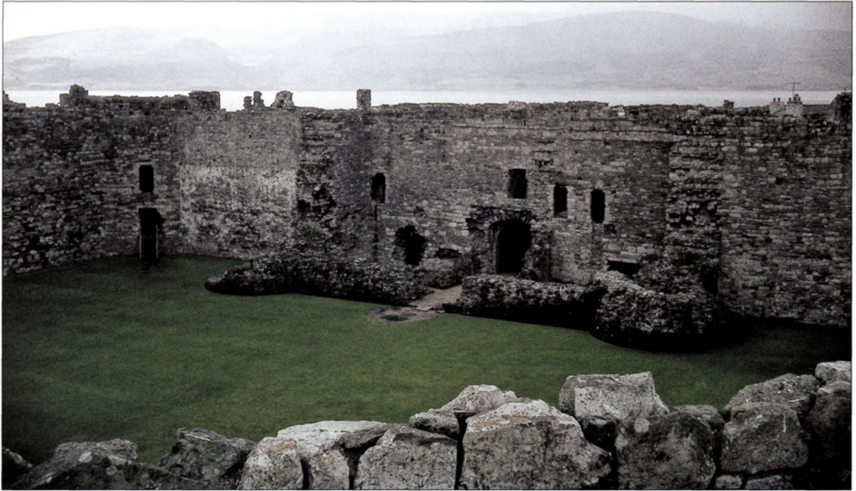
The inner side of the South Gatehouse at Beaumaris. The walls may never have risen much beyond their present height.
