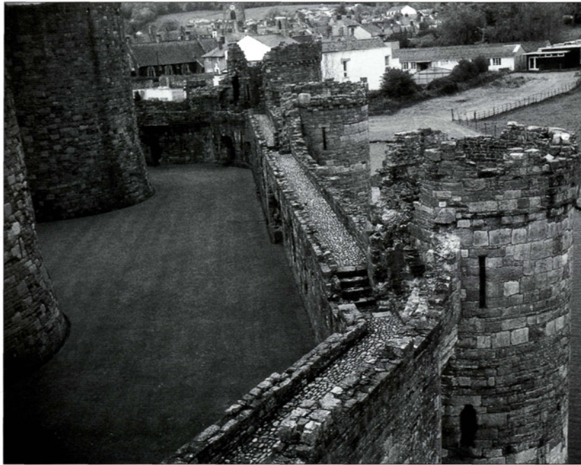
Towers 13 to 15 on the outer curtain at Beaumaris, with the battered plinths of the inner towers clearly visible.
