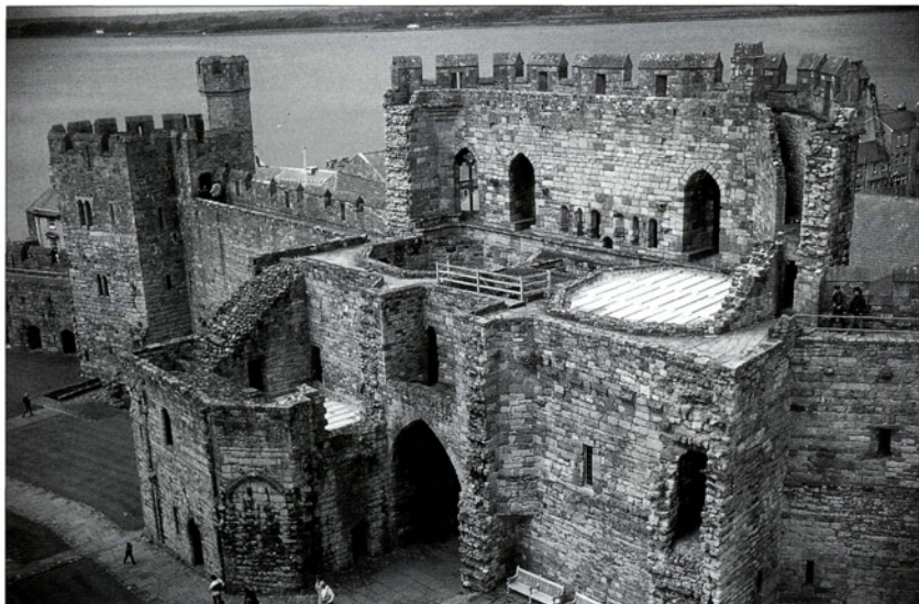
The rear of the King's Gate at Caernarfon. The toothings for adding stonework to the vertical wall ends suggest it was never completed. The gate passage opens into what would have been a right-angled turn with portcullis groove visible on the corner to the right of the small doorway. Above the gate passage was a chapel, and on the floor above a hall, marked by the large windows. The two blocks of three embrasures at the centre of this wall are multiple arrow loops, each block feeding one loop. At far left can be seen ground-level embrasures serving single arrow loops.
